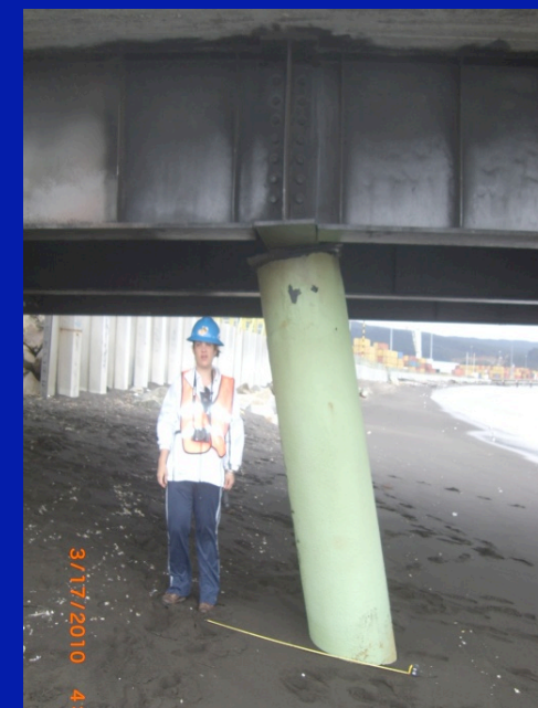
Coronel : a) Lateral Spreading/Settlement, b) Sediment Ejecta/Sinkholes, & c) Pile Damage
